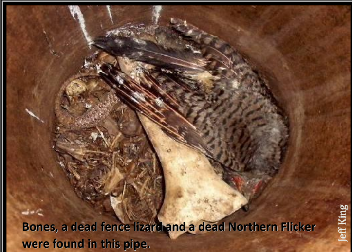
50 year old uncapped irrigation vent pipe.
